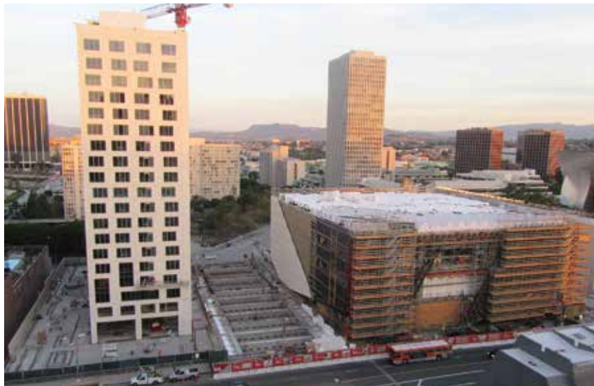
Field trips include site visits to buildings underway, including these three adjacent projects in downtown Los Angeles: the Grand Avenue Apartment tower, the Grand Avenue bridge park, and the Broad Museum.
